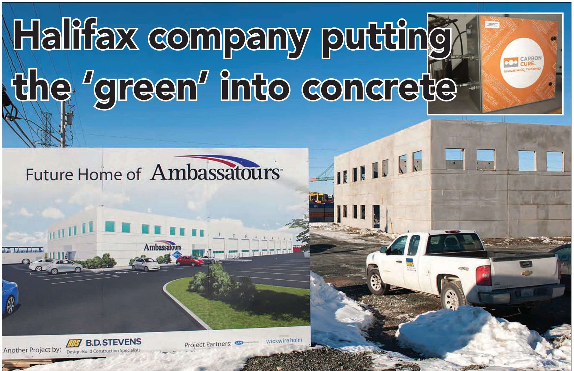
The new home of Ambassatours in Halifax was the first building in the world to be made with ready mix concrete products using CarbonCure. Inset, the CarbonCure system injects liquefied CO2 from a pressurized tank into the concrete mix. - Submitted photos
